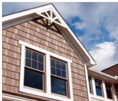
Double-hung windows with half-colonial grilles
